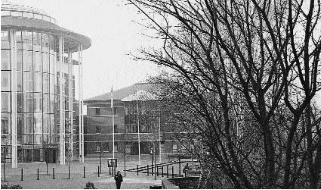
Figure 4.15 Canalside development, Nottingham: The Courts.
